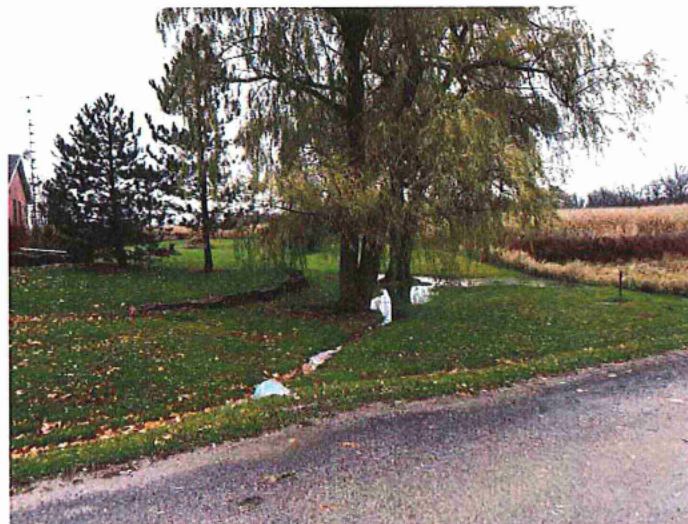
(1) From Con. Road 2 facing north; Drainage on neighbouring property.
