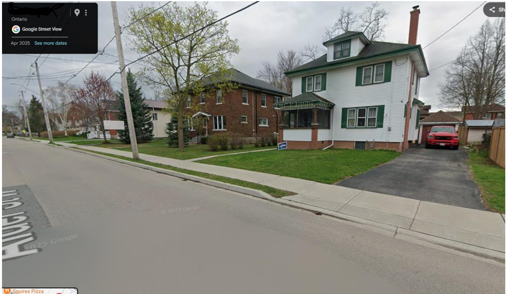
Figure 1 Alder Street West Photo - View from the road of the property, curb, and driveway
